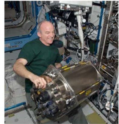
NASA astronaut Jeffrey Williams, Expedition 22 commander, installs a Urine Processor Assembly / Distillation Assembly (UPA DA) in the Water Recovery System (WRS) rack
